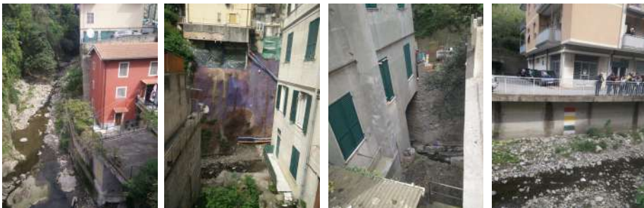
Figure 2 - Examples of constructions in the river-bed observed during the excursion along the Ferreggiano river
